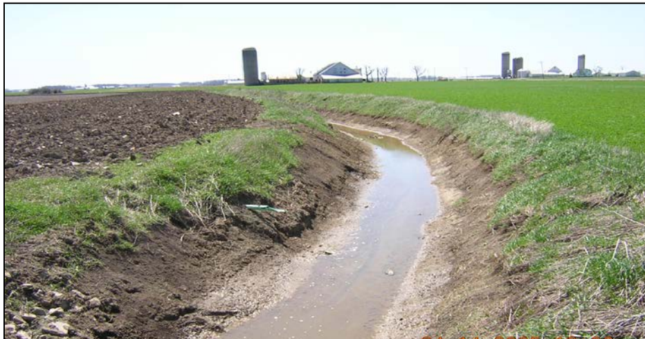
Figure 5: Channel maintenance that "dips out" bottom sediments and removes bank vegetation to reestablish the trapezoidal geometry.
