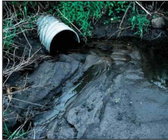
Figure C4: Sediment deposition impacting performance of subsurface drainage system. (Photo: NRCS Gallery)
