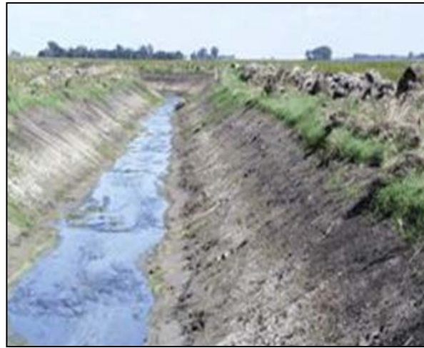
Figure C7: The same ditch seen in Figure 6 after the maintenance activity.
