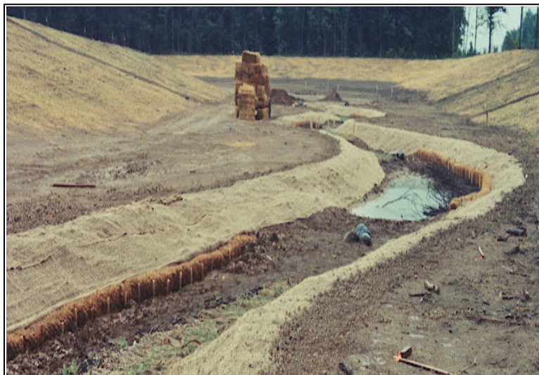
Figure C14: A natural channel design during construction.
