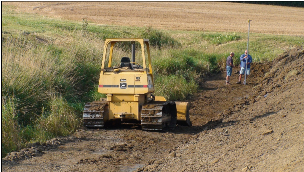
Figure C25: Construction of a bench wide enough to accommodate a bulldozer for any maintenance needs, if necessary.
