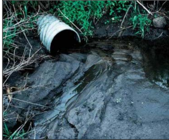
Figure 4: Sediment deposition impacting performance of subsurface drainage system. (Photo: NRCS Gallery)
