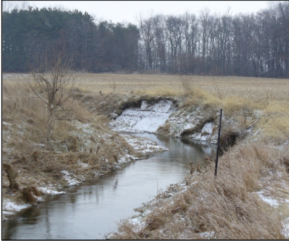
Figure 3: Mass wasting of a bank from erosion of the toe making the banks steep and prone to failure.
