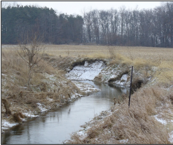
Figure C3: Mass wasting of a bank from erosion of the toe making the banks steep and prone to failure.
