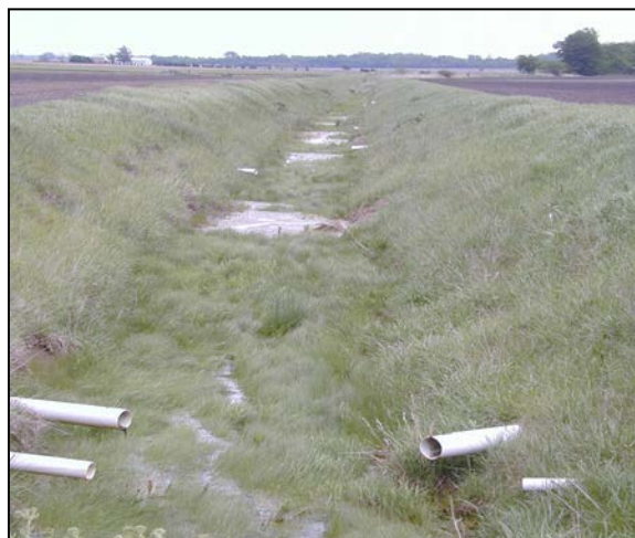
Figure C2: Subsurface drains outletting to a typical surface drainage channel in the North Central Region of the United States.
