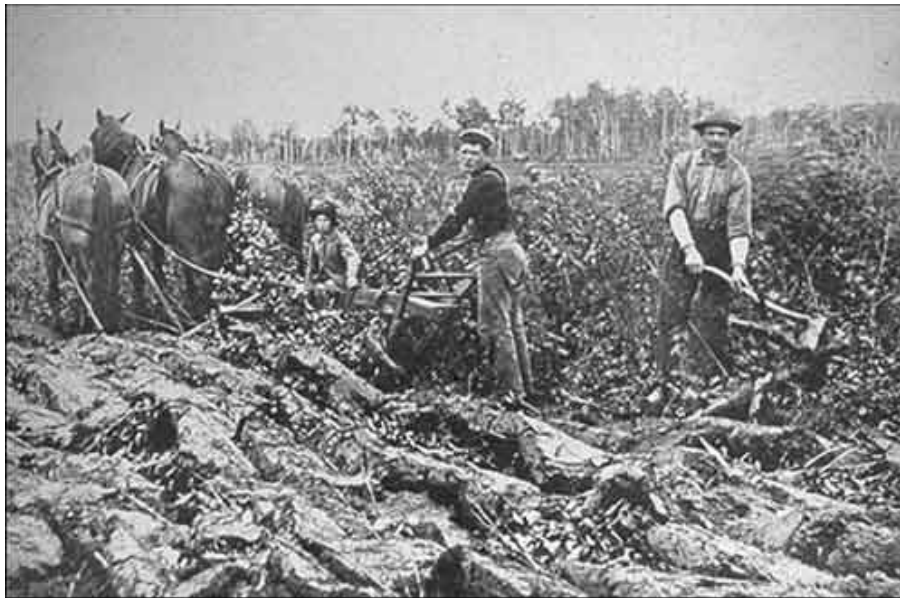
Figure B5. Land clearing preceded cultivation during early American settlement.
