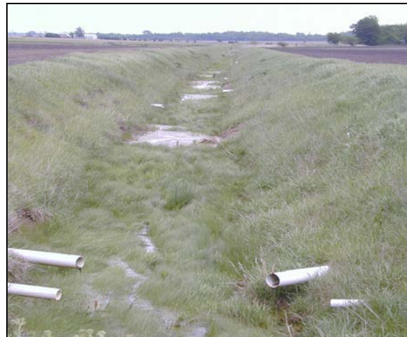
Figure 2: Subsurface drains outletting to a typical surface drainage channel in the North Central Region of the United States.
