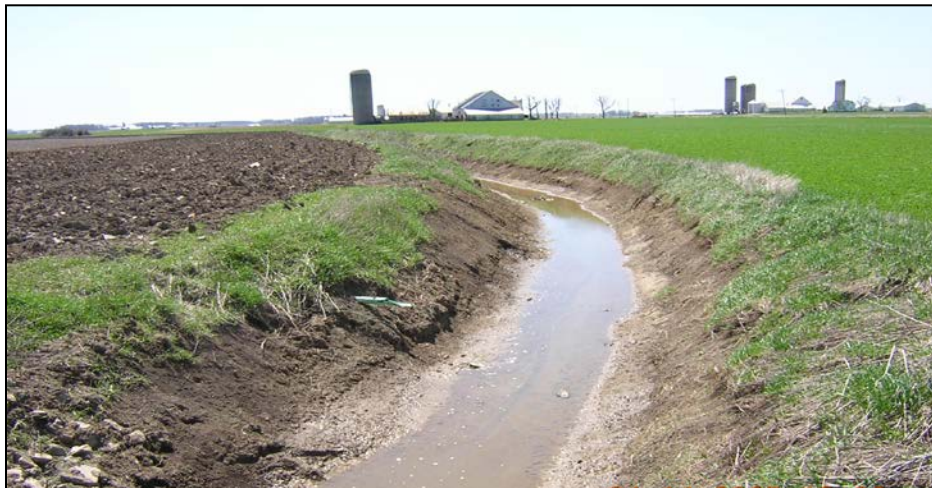
Figure C5: Channel maintenance that "dips out" bottom sediments and removes bank vegetation to reestablish the trapezoidal geometry.
