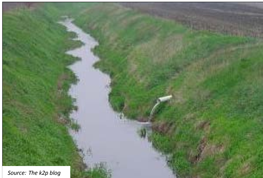
Figure B9. An over-sized open ditch to accommodate subsurface tile outlets.
