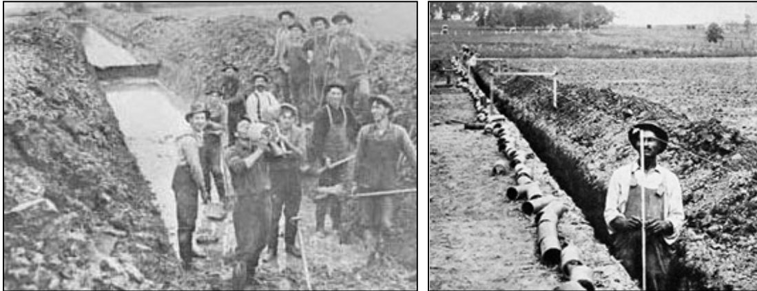
Figure B1. Surface ditching and subsurface drain tile done by hand in the early 1800s.
