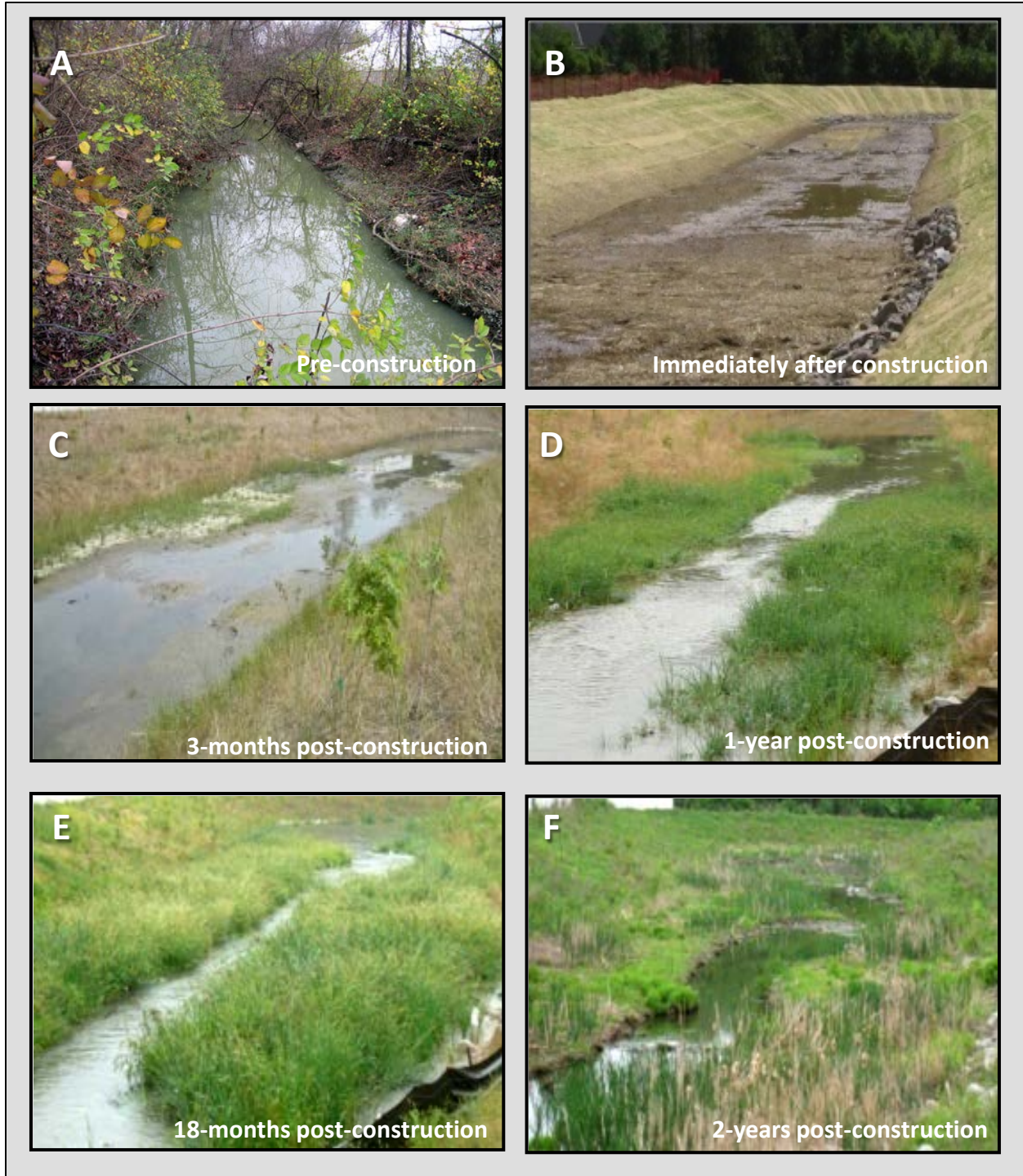
Figure C13: Time series photographs of Beem Ditch in Columbus, Ohio. A) Pre-construction, B) immediately after construction, C) 1-year post-construction, D) 1-year post-construction, E) 18-months post-construction, and F) 2-years post-construction.
