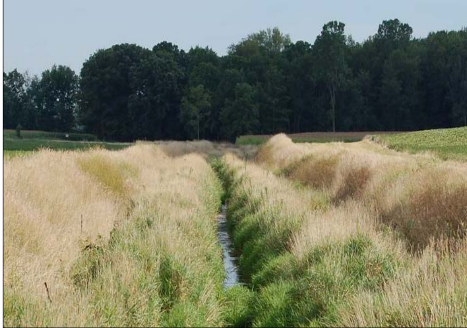
Figure B17. A stable two-stage channel in Hillsdale County, Michigan, six years after construction.
