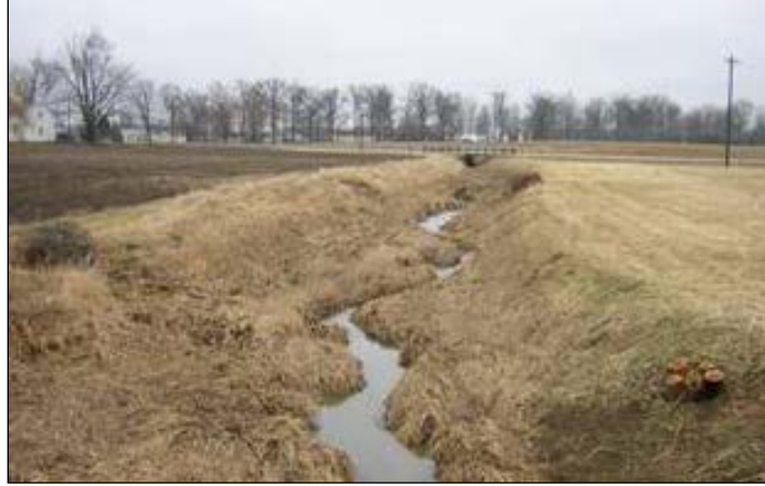
Figure B12. An agricultural drainage ditch with vegetated benches and a meandering inset channel.
