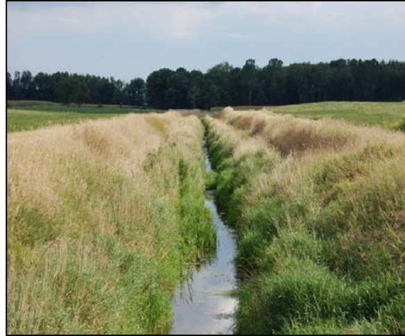
Figure C9: Crommer Ditch two-stage reach approximately 6-years after construction.
