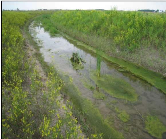
Figure C11: Self-formed stream at the tributary to Muddy Creek near Kansas, OH. Photograph is shortly after construction.
