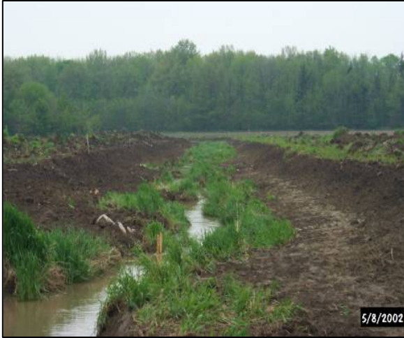
Figure C8: A tributary channel to Bull Creek in Wood County, OH during two-stage channel construction.
