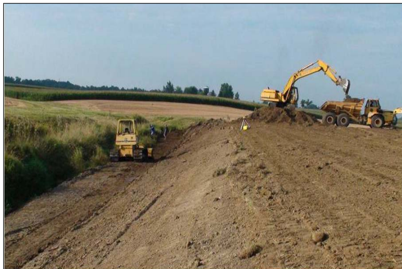
Figure B16. Construction of a two-stage ditch leaves the inset channel intact and “pulls back” the benches to a width that is a multiple of the bankfull channel width or wide enough to accommodate small machinery.
